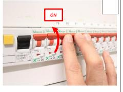
**2.** If you have external circuit breakers. Check that all the breakers are in **ON** position. **IMPORTANT!** Call an electrician if the breaker trip again
