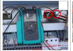
**7.** Measure ~volts on all heaters (700 series = 10 heaters and 800, 900 = 14 heaters) there Should be **no voltage**
