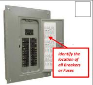
**1.** In your **electrical circuit box**, check and identify the position of all the external circuit breakers or fuses for the oven
